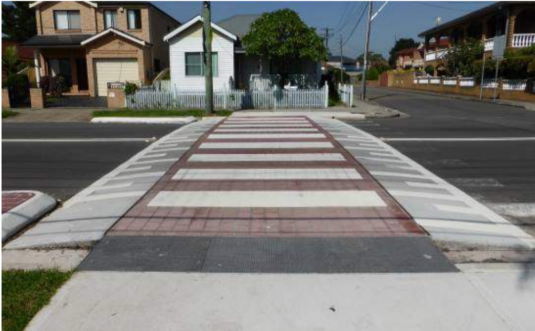
Figure 30: Raised pedestrian crossing
